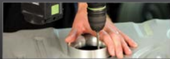
Use installation ring to locate mount holes
