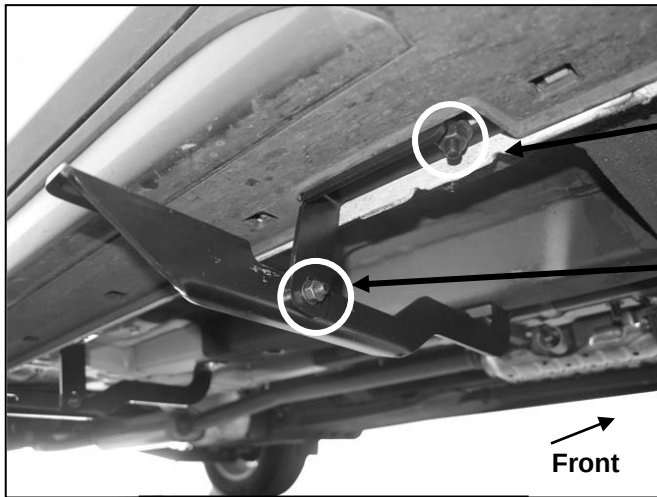
(Fig 7) Passenger side Front Support Bracket installed
