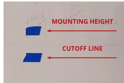
10. Mark the mounting height on the wall or garage door using tape.
