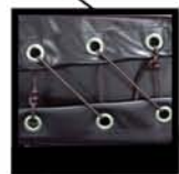
Grommets away from frame eliminates contact wear
