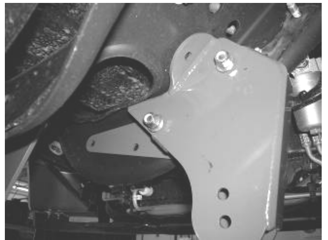
Passenger Side I-beam Bracket Driver I-Beam connection point
