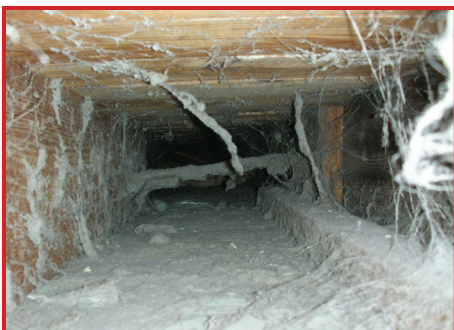
Inspection of hard-to-reach and hard-to-see areas
