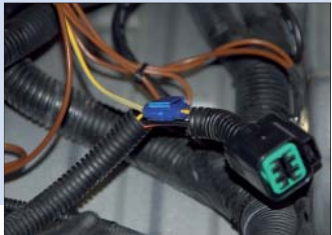
Driver side: Yellow cable Passenger side: Yellow cable
