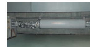
Seismic Isolation Oil Dampers
