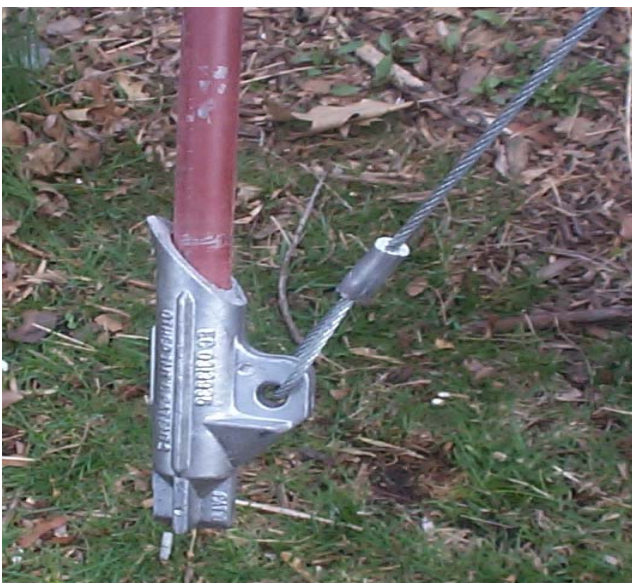
Drive Rod inserts into Anchor Head
