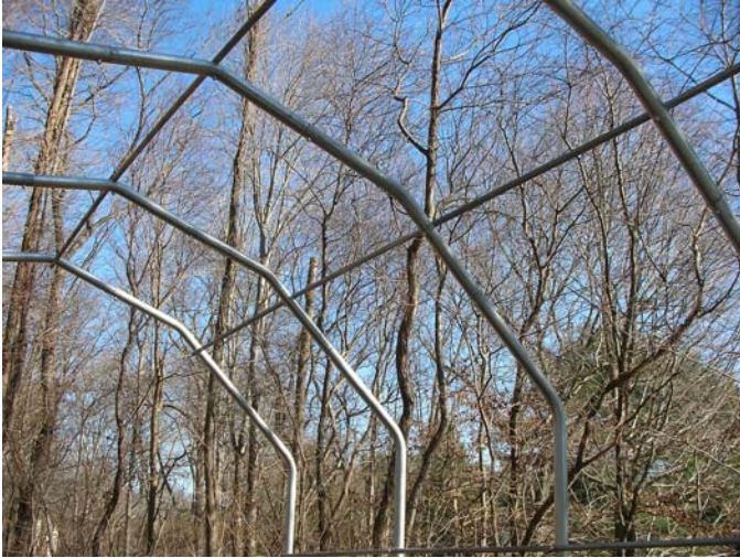
Side & Top Cross Rails between Arch Assemblies
