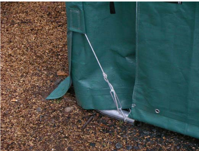
Main Cover Turnbuckle secured to Base Foot
