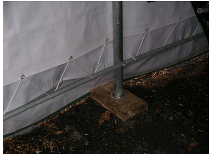
Lace rope through grommets and around Base Cross Rails
