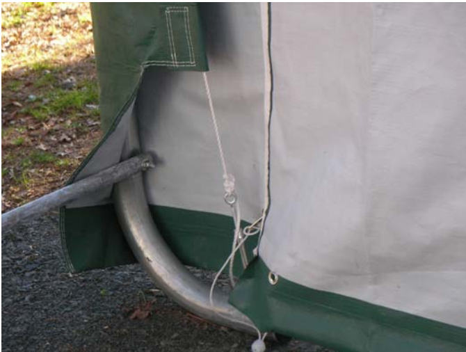
Door Turnbuckle Attached to Base Foot
