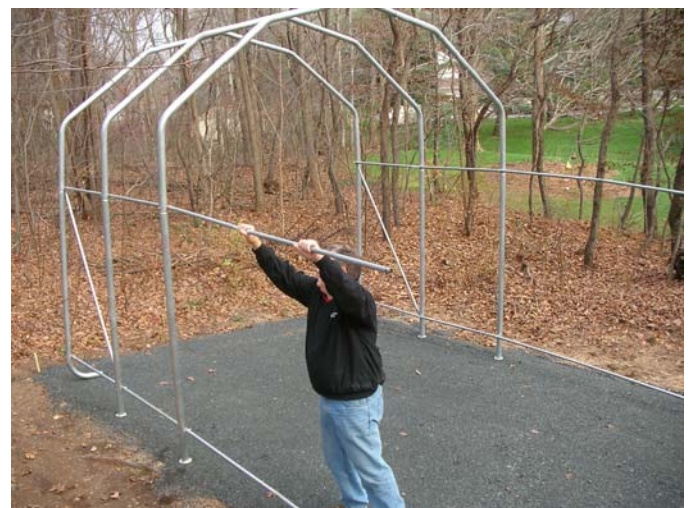
Add Cross Rails in preparation for adding Arch Assemblies
