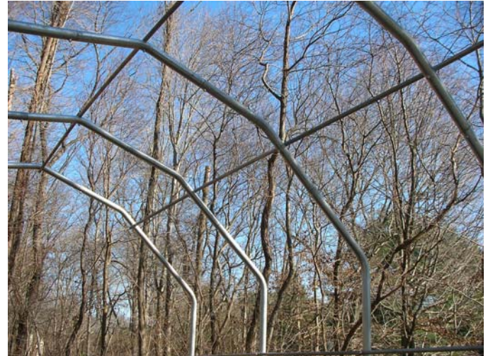
Side & Top Cross Rails between Arch Assemblies
