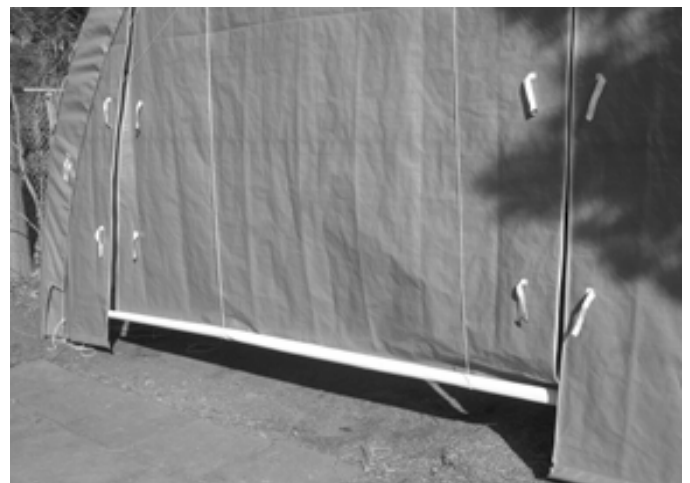
Place the two-piece rail into the base pocket of the doors for weight and rigidity to roll easily.
