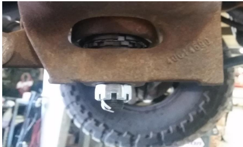
Figure 14. Cotter Pin Installed
