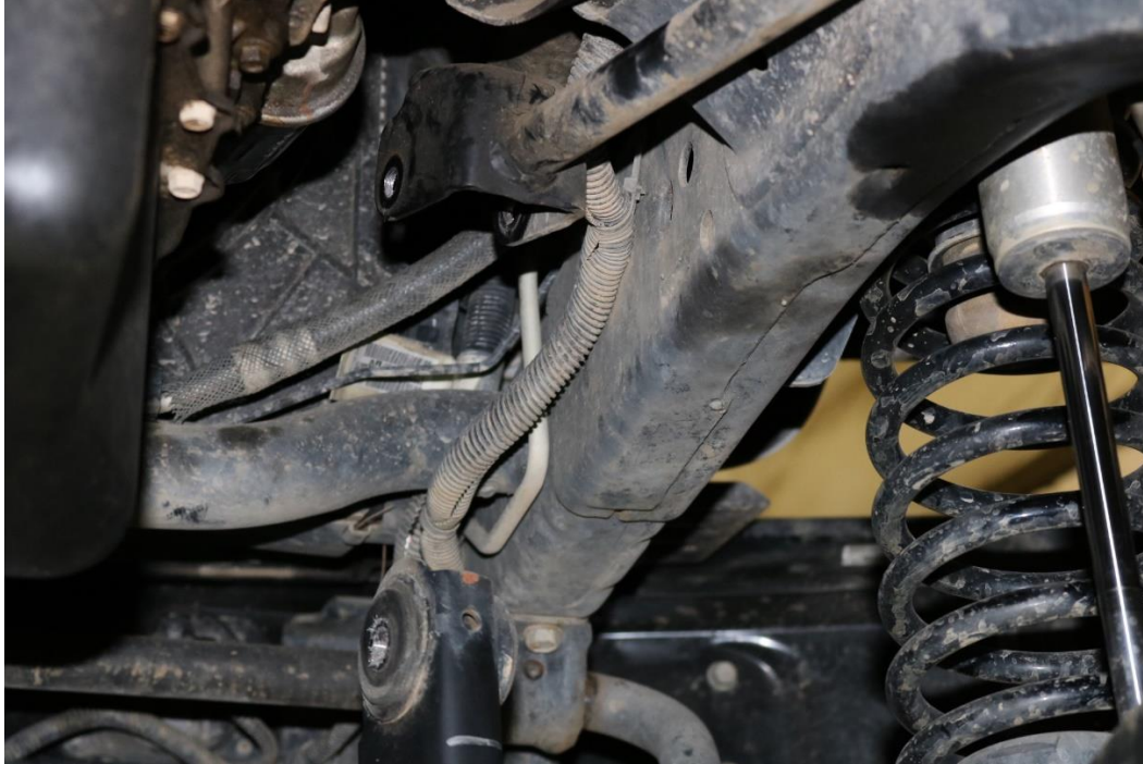
Figure 1. Right Side Front Upper Control Arm Rotated Up
