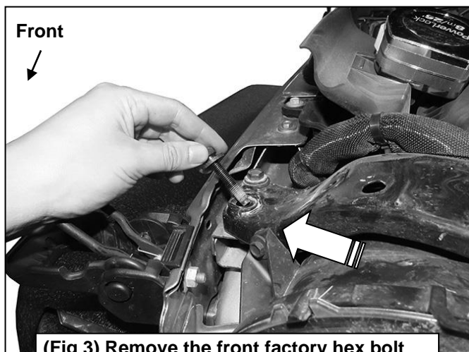
(Fig 3) Remove the front factory hex bolt from the top of the radiator support (arrow)
