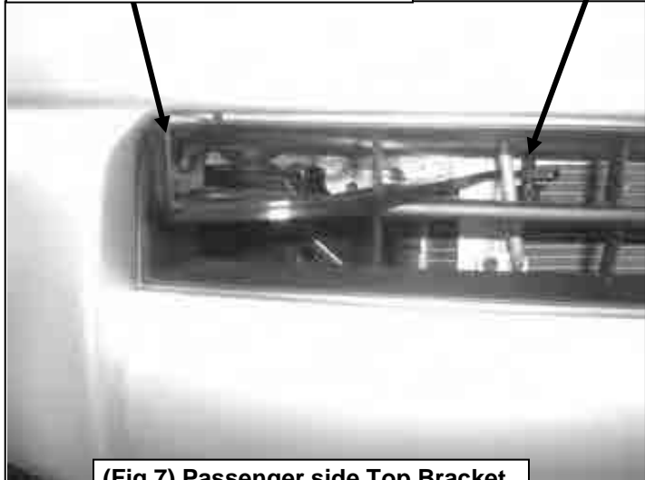
(Fig 7) Passenger side Top Bracket installation through grille opening
