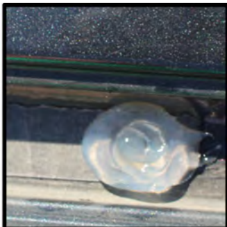
Next apply silicone over the holes
