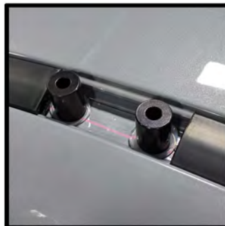
Then place the spacers over the holes and silicone and press down making sure a good amount extends around the edge
